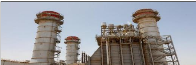
Amman East Power Plant
