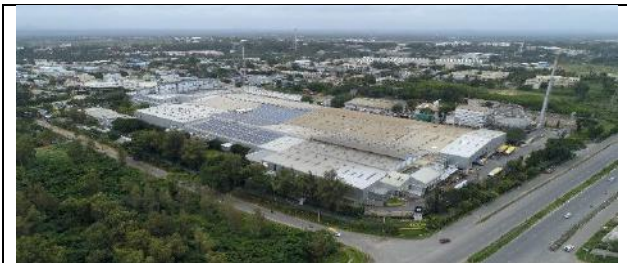
JK TYRE & INDUSTRIES LTD., VIKRANT TYRE PLANT
