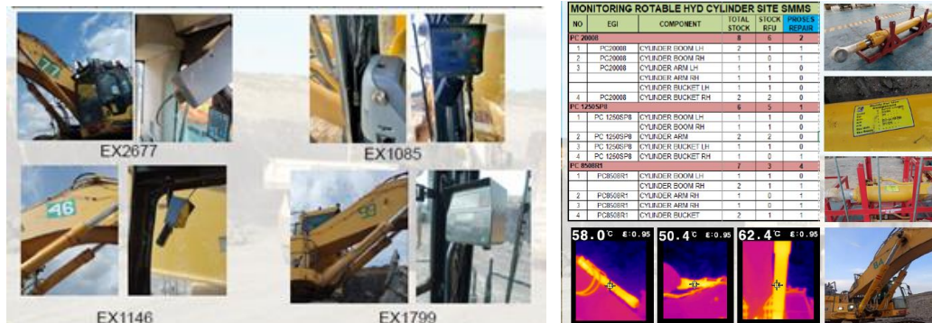
Figure 19. POCYS and loader cylinder monitoring
